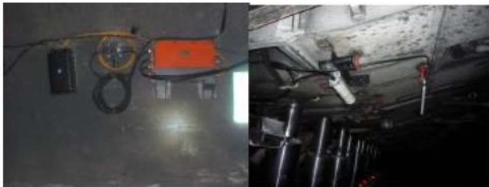
Fig.4. Base station installation on site
